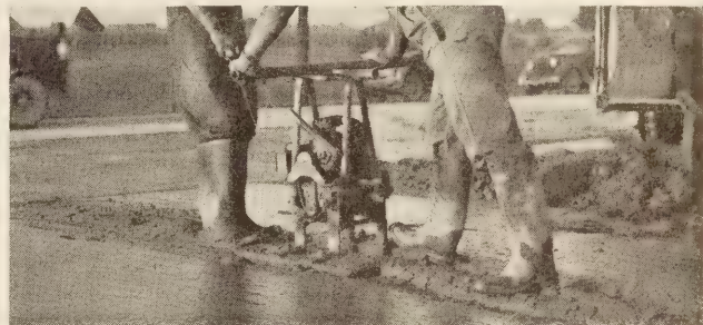
FIGURE 15.—VIBRATORS USED AROUND TYPE III JOINTS. UPPER, VIBRATOR USED ON EAST PROJECT; LOWER, VIBRATOR USED ON WEST PROJECT.
